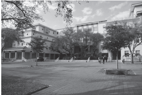
Figure 5563-1. Seering Administration Building at Ringlin in Sarasota 2009.
