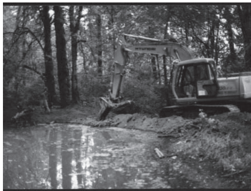
Figure 675324-1. David Parker makes a dam at Mtn Grove Forest with shovel & excavator.
